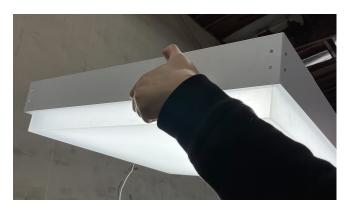
Install the last frame of the SMK to complete the installation. Check all the corners to ensure the alignment as well as proper installation.
