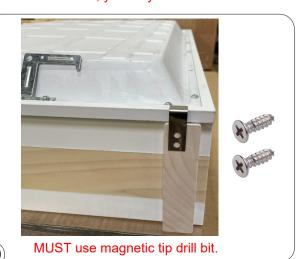
Place the clips at each corner, use 2 screws per clip to fix altogether.
