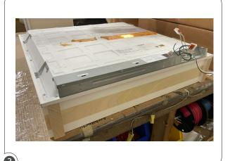
Place the flat panel (2x2 or 2x4) on top and position the corner.
